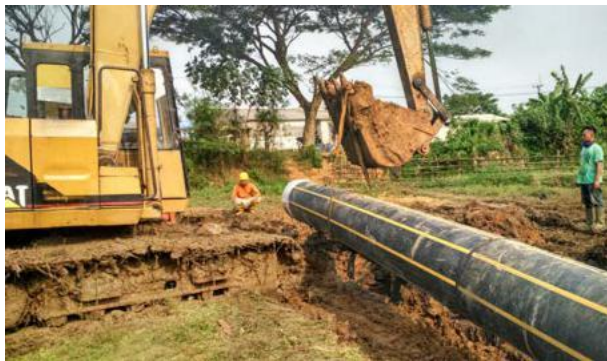
(710mm pipe, water treatment for modern industrial estate)
