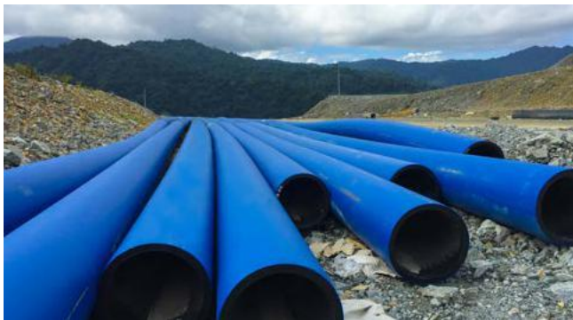
(315mm pipe, water distribution)
