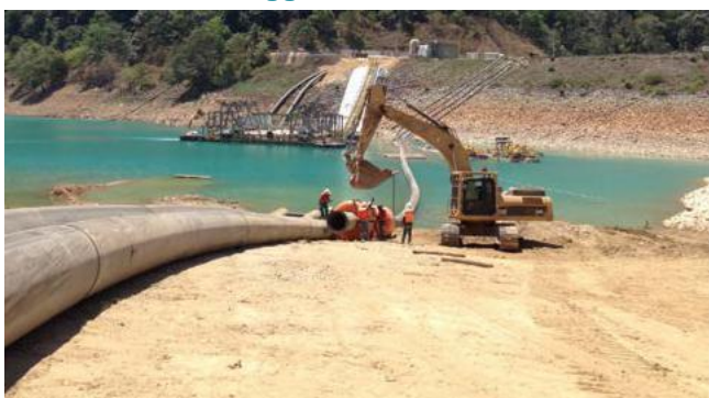
(1000mm pipe, dewatering systems project)
