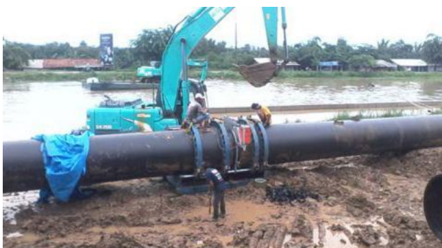
(1200mm pipe, siphon water project)
